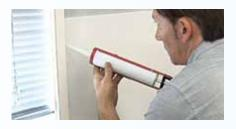
PANEL INSTALLATION: Seal the joints with neutral cure wet area silicone. Once gap is filled, remove excess silicone using a soft flexible plastic spatula.
