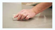
PANEL INSTALLATION: Scuff the rear surface with coarse scouring pad or 240 grit sandpaper.
